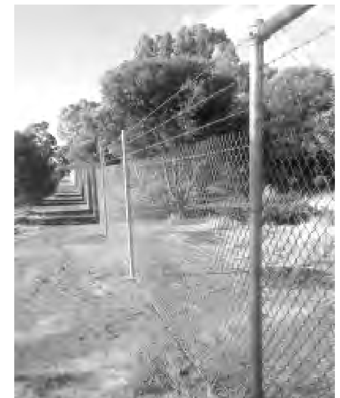
New fence at Charlton Landfill site
