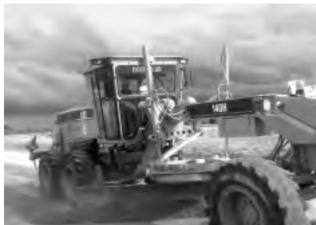
Grader crew at work maintaining shire roads.
