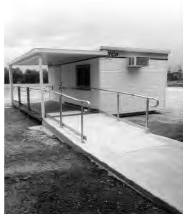
New portable office building at the Wycheproof Saleyards
