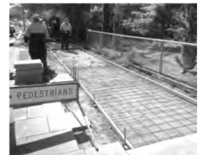
Concrete Crew carrying out footpath Capital Works in Broadway, Wycheproof.
